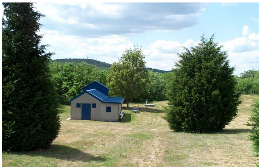
Figure 37: Drinking water pumping station Klariči
