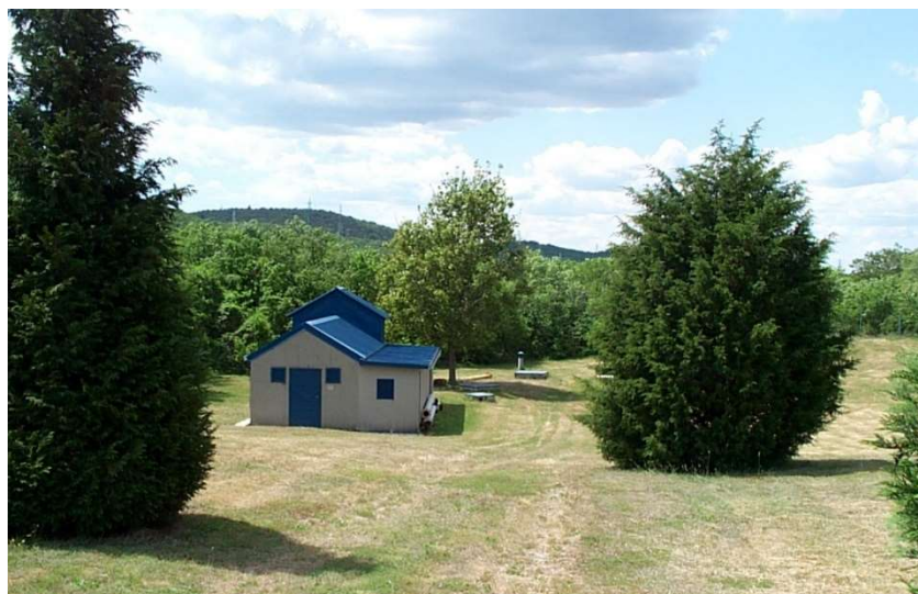
Figure 37: Drinking water pumping station Klariči
