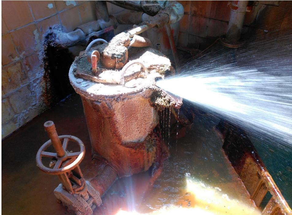
**Figure 7.2.** Uncontrolled hot water flow leakage @50°C from the ‘Jafre’ well head (photo: August 2017).
