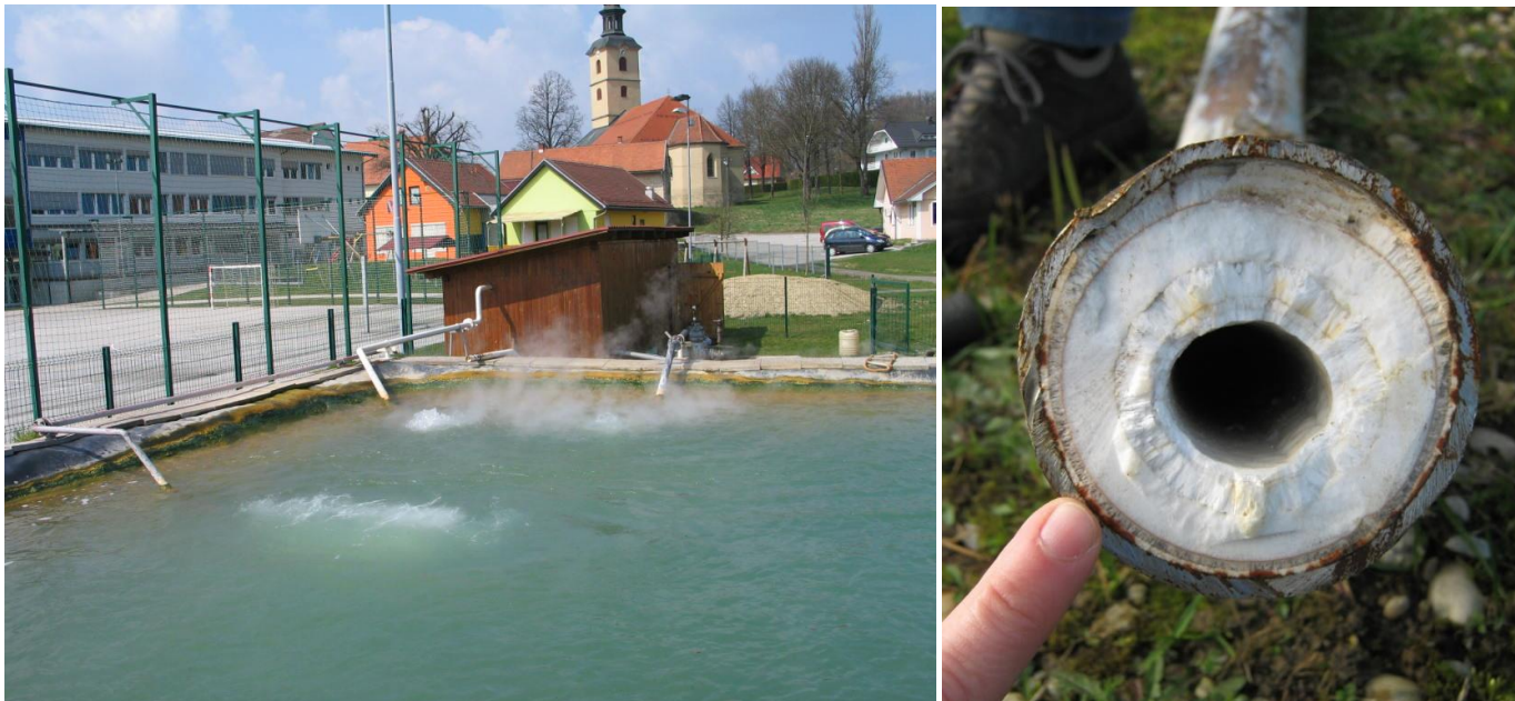
Fig. 1. Left: Cooling pool at the wellhead of Be-2 (see it right of the wooden house) where pulses due to degassing are evident. Right: Thermomineral water has high scaling potential and even though an inhibitor was injected in the well there was lot of carbonate scaling in the pipes.
