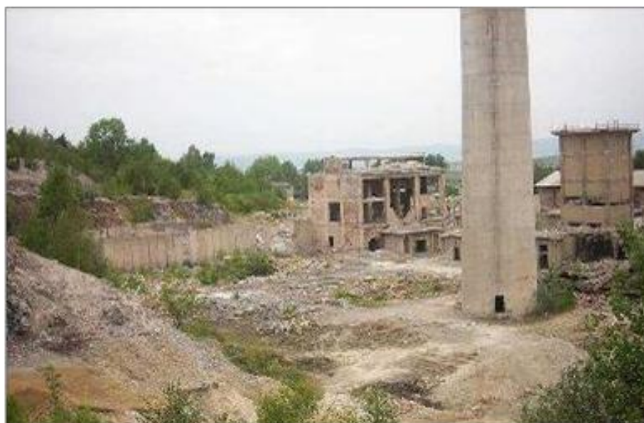
Figure 3: The ruins of the former nickel smelter in the Szklary (Lower Silesia, SW Poland)
