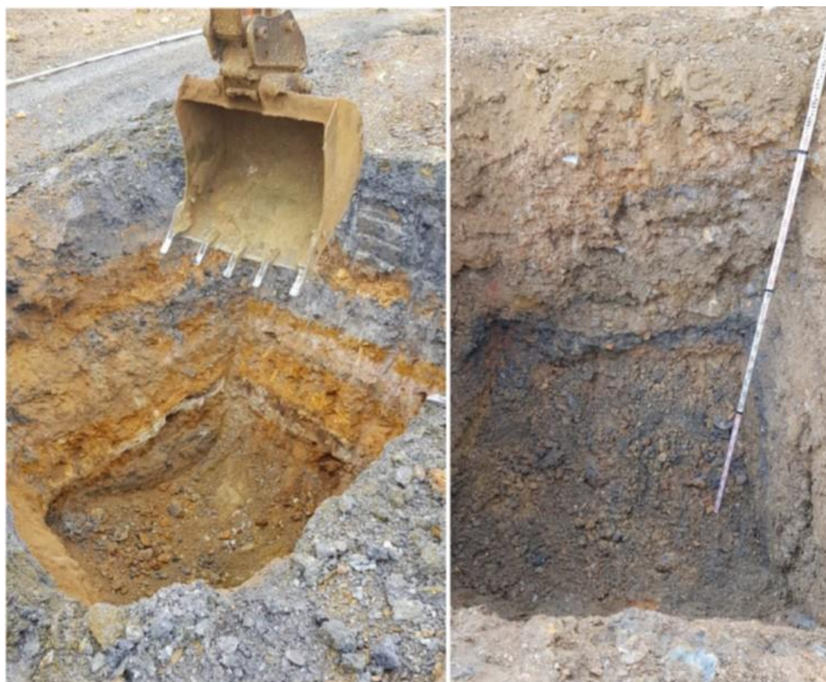
Figure 6: Example trial pit through the spoil heaps at Avoca. The measuring stick on the right-hand photo is 4 m long.
