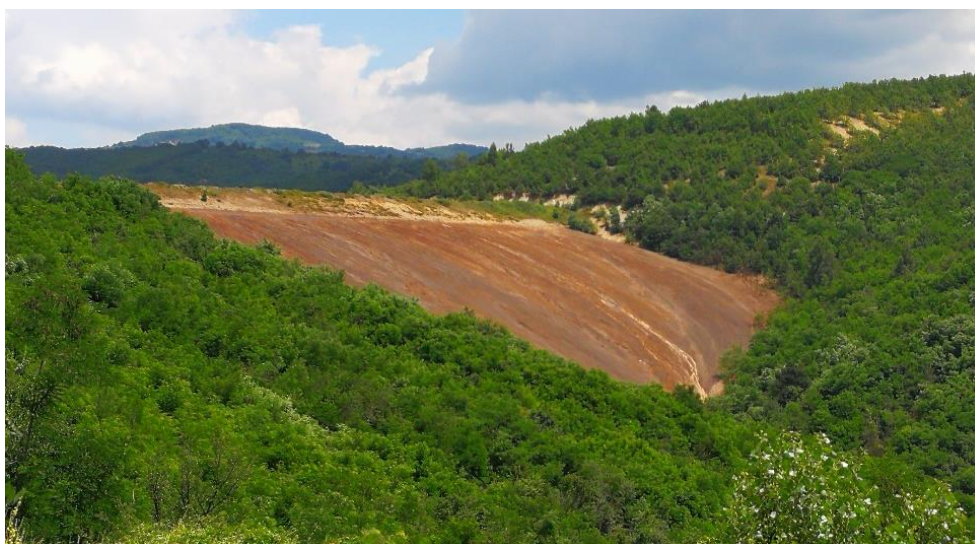
Figure 7: Front of the dam of the Kelmendi Tailings pond
