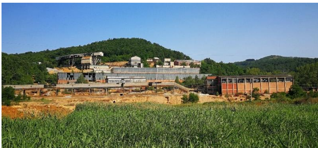
Figure 13: Flotation plant at Kishnica
