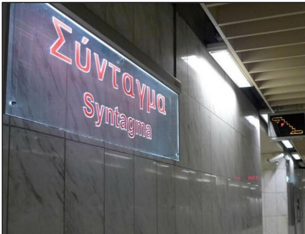
Syntagma – Metro Station: Cladding with Volakas marble.
