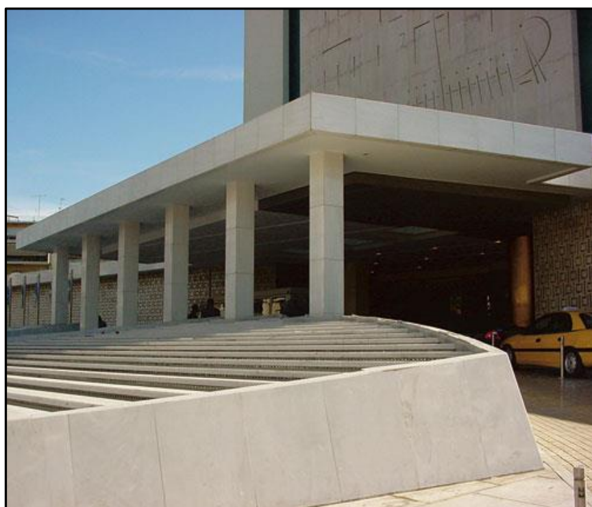
Hilton Hotel Athens: Wall cladding with Thassos Limenas marble.
