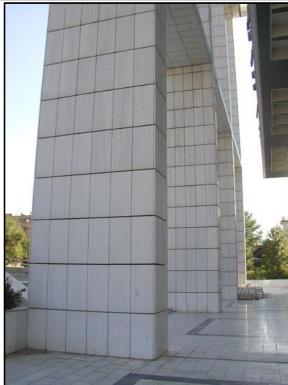
County Court-Athens: Cladding with Thassos Limenas White.
