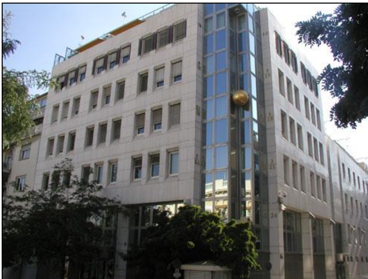
Building of the German Embassy in Athens: Wall cladding with Thassos Limenas marble.
