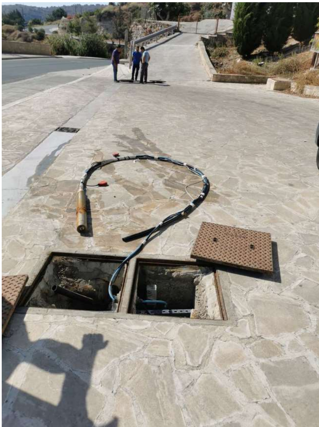
Description: Paving with Mitsero limestone.
