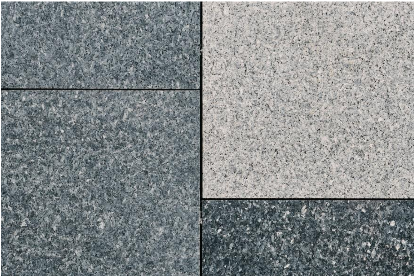
Façade with different surface treatment (photo Lundhs/Morten Rakke)
