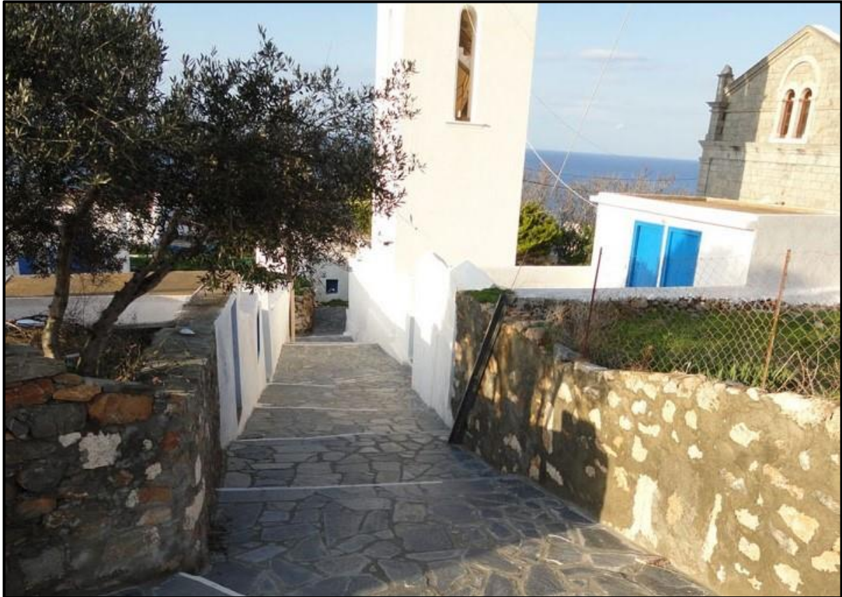
Paving of roads and footpaths on the island of Kassos with polygonal Karystos slates.
