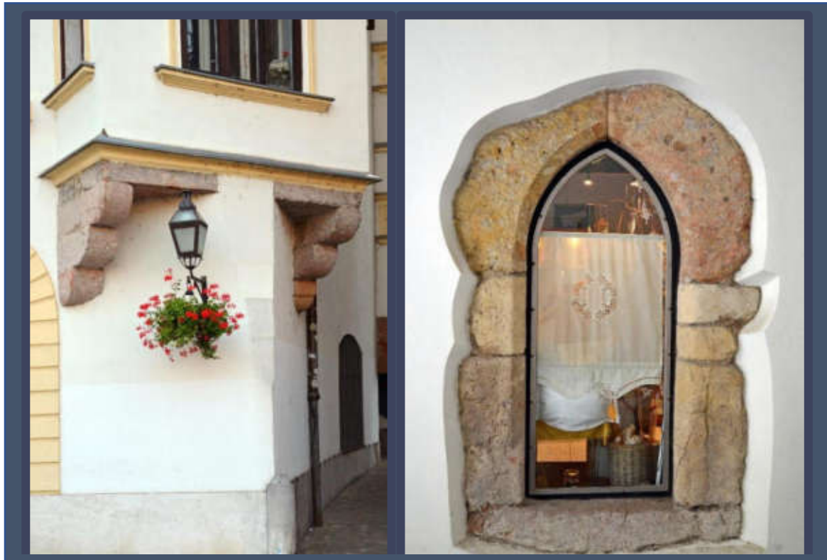
Škofja Loka conglomerate preserved as decorative architectural elements in renovated buildings in Ljubljana.
