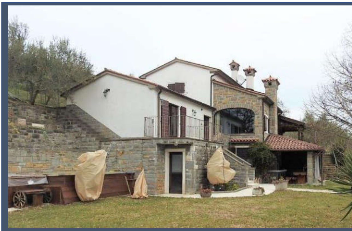
Private residence in Puče in Slovenia Istria built with blocks of Jelarji sandstone.
