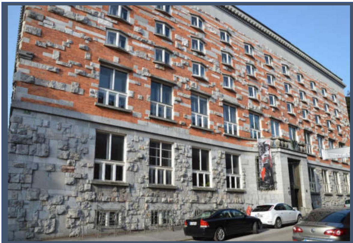
Podpeč limestone blocks in the Plečnik's National and University Library in Ljubljana
