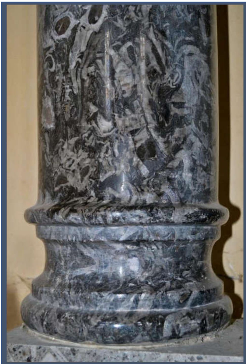
Altar pillar made of Kazlje limestone in St. Elija Parish Church (1823) in village Kopriva in the Kras region.
