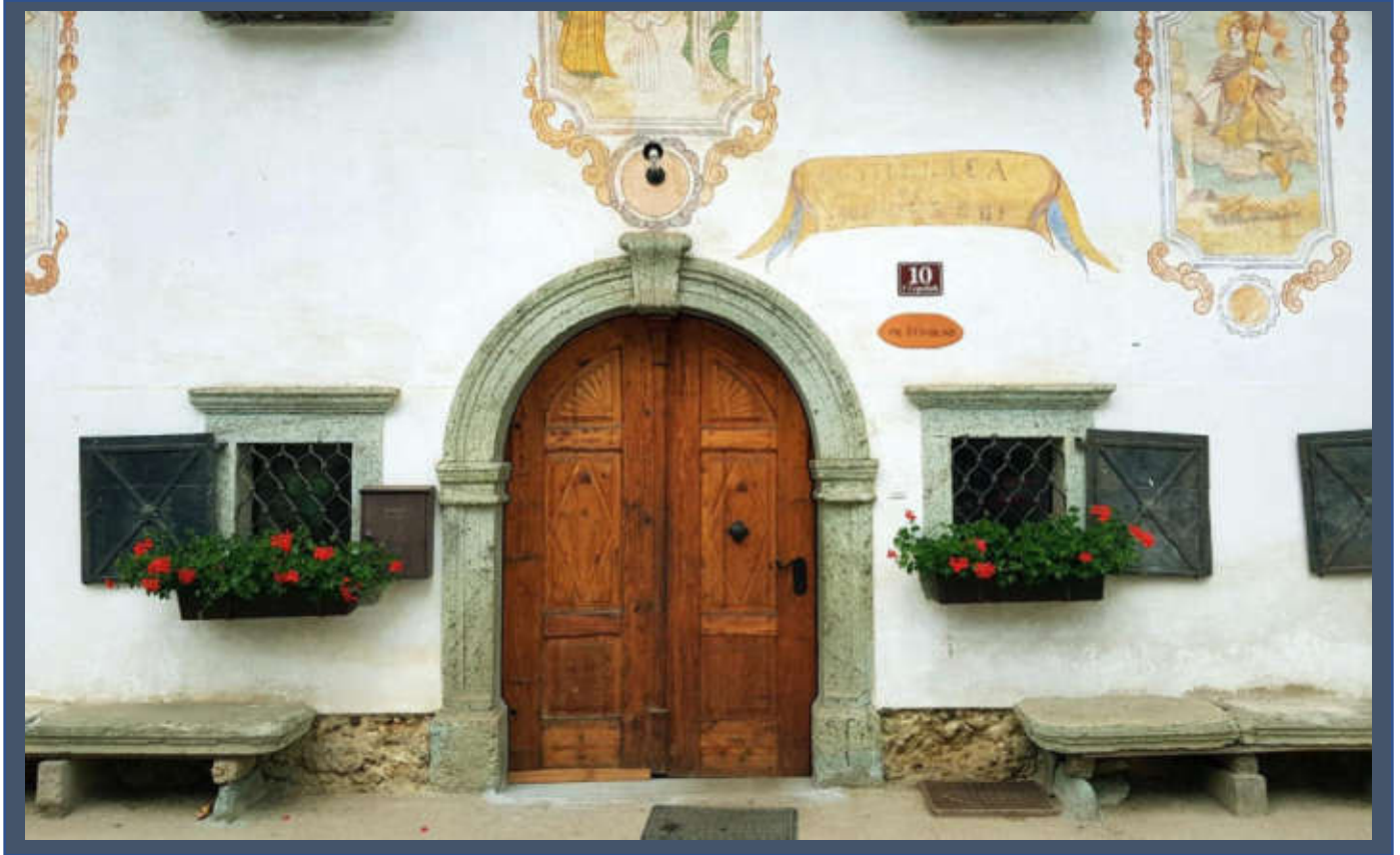
Country house in Zgornja Besnica with entrance portal, window frames and benches made of Peračica tuff.
