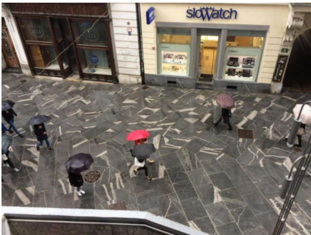
The Čopova street in Ljubljana paved with Pohorje granodiorite with decorative aplite-pegmatite veins.
