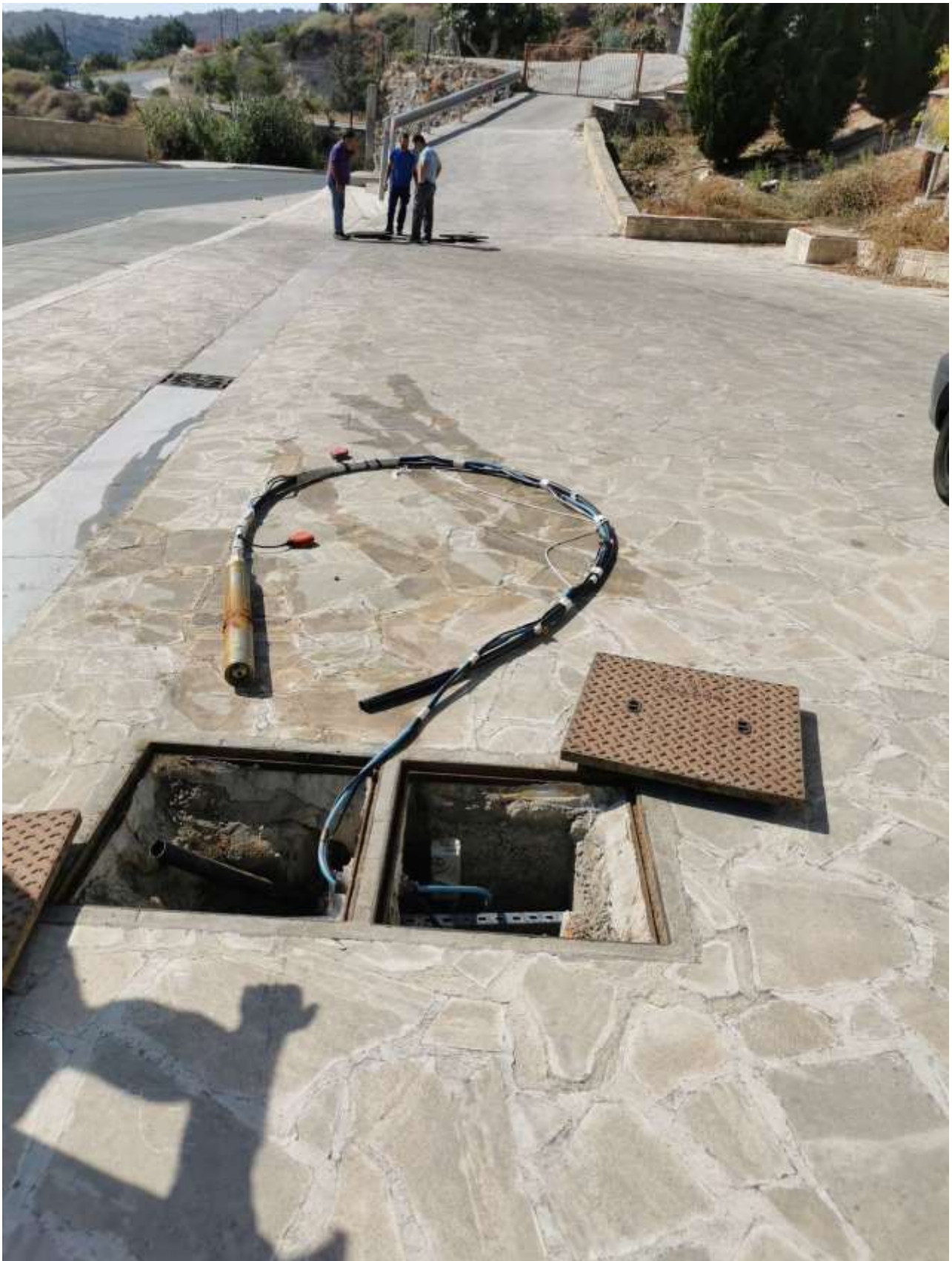
Description: Paving with Mitsero limestone.
