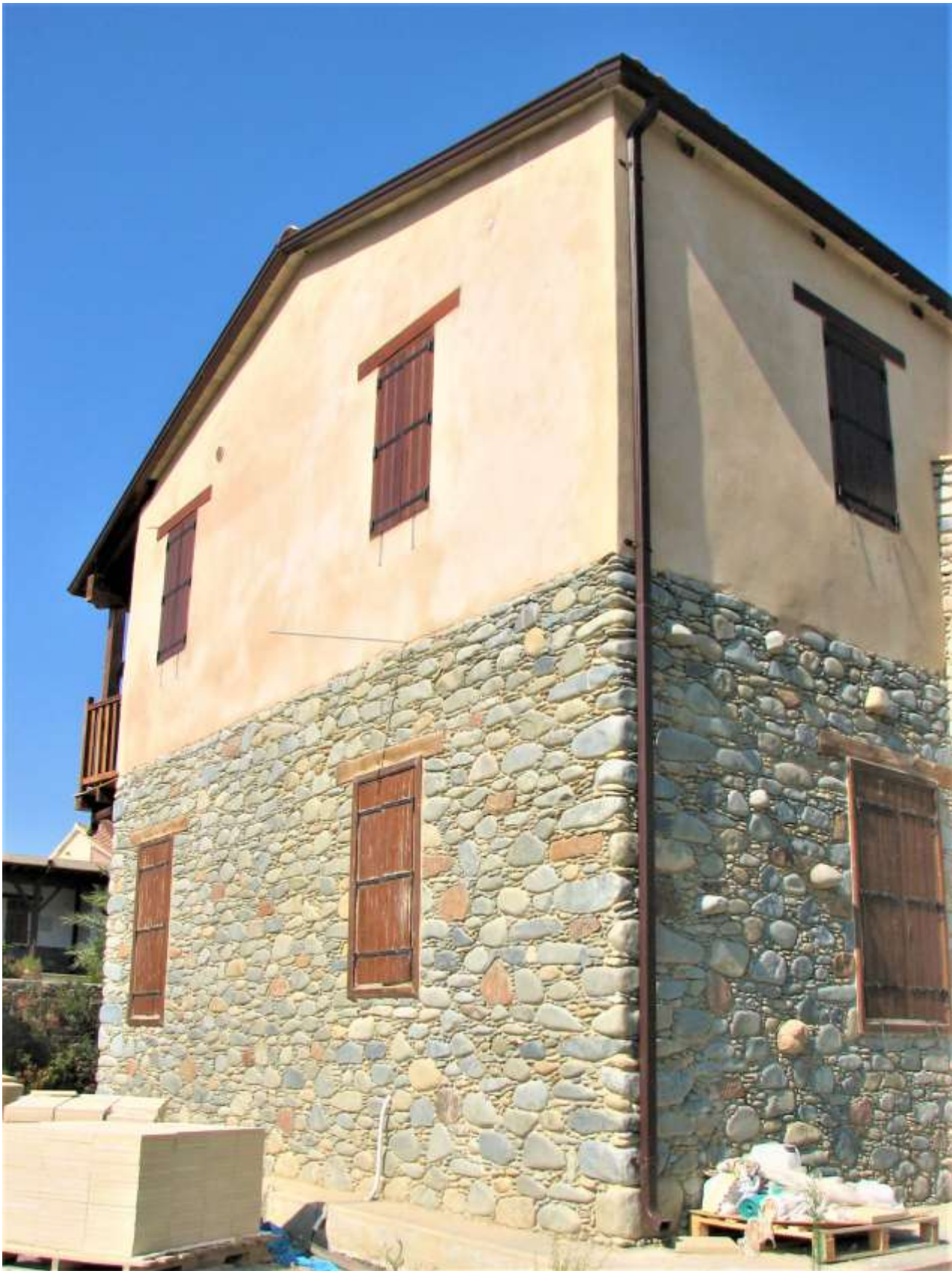
Description: Description: House clad with diabase and other igneous rocks.
