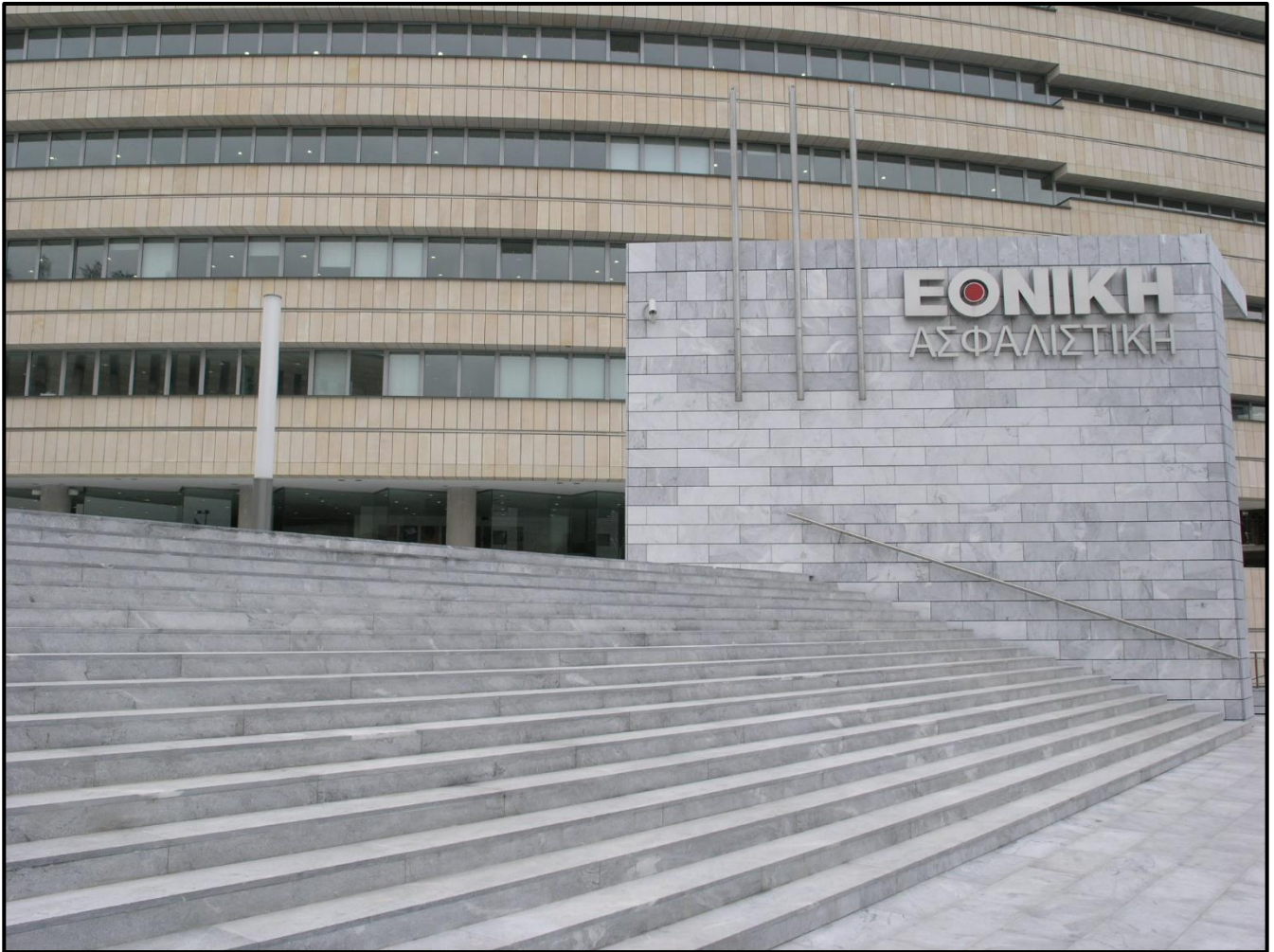
Building of Ethniki Hellenic General Insurance Company: Exterior flooring, stairs and cladding with Aliveri Grey.
