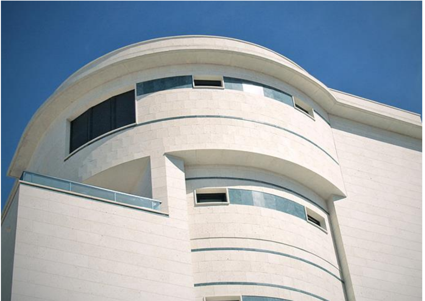
Cladding of modern building. Image source: www.gruposanmarino.com
